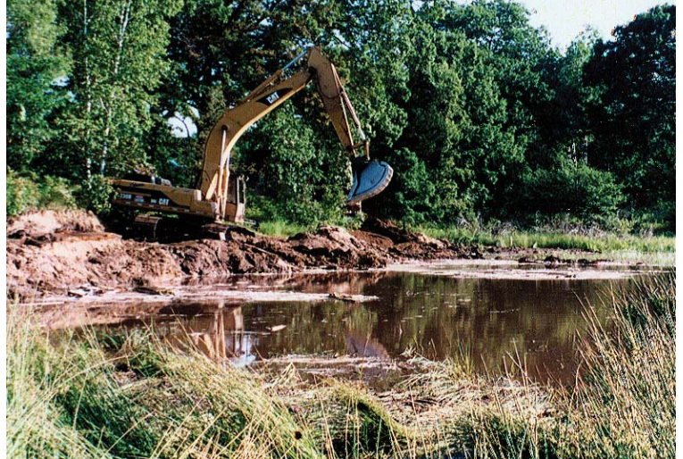
Figure 2. Dragline (backhoe) Dredging
