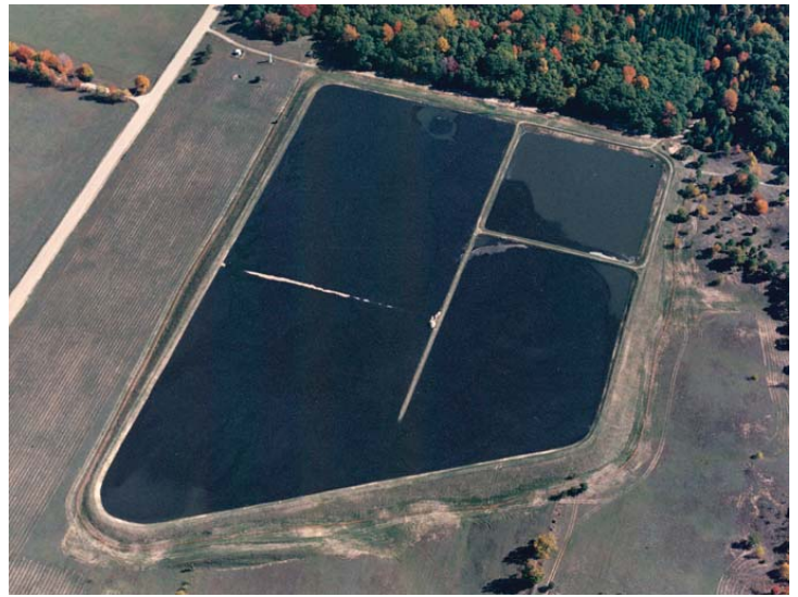
Figure 4: Dredged sediment disposal cell
